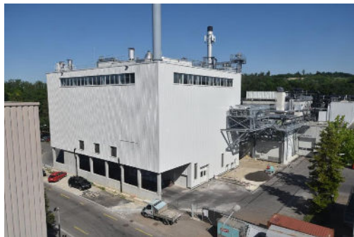
MBM Gasifier Plant 18 MWth steam + 2 MWe. Lyss, Switzerland
