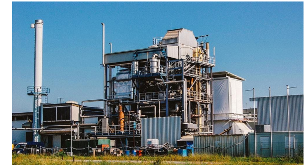
Indirect gasification plant in Güssing (Austria)
